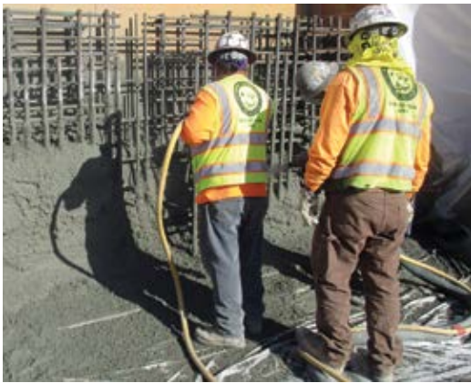
Fig. 2: Crew shooting preconstruction test panel
