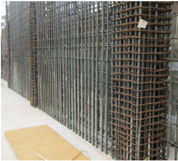
Fig. 9: Heavy reinforcing layout for a parking garage wall
