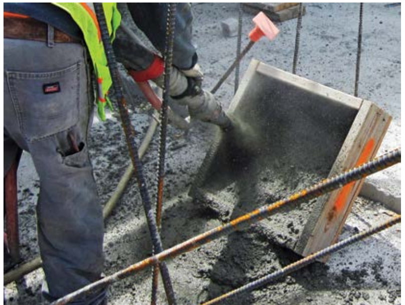
Fig. 11: Typical daily wet-mix shotcrete production panel
