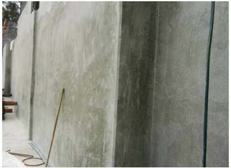
Fig. 10: Completed parking garage wall
