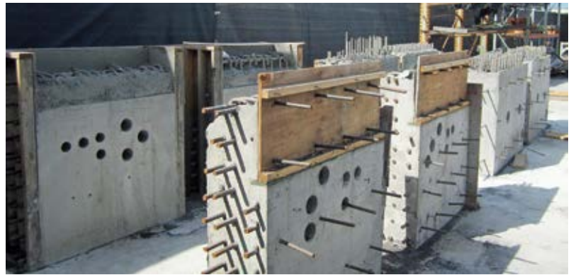
Fig. 3: Preconstruction test panels have been stripped, cored, and inspected
