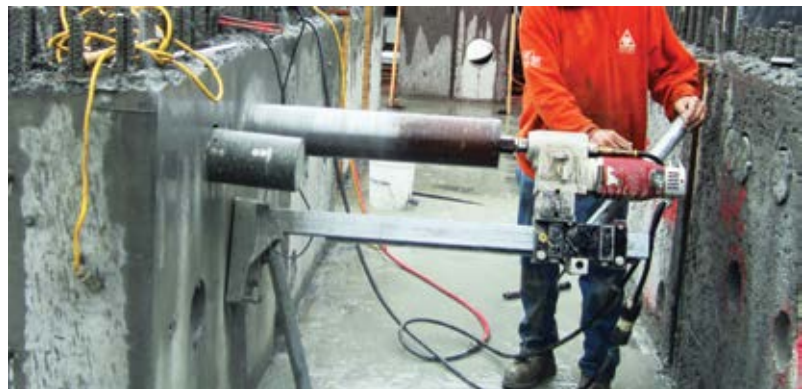
Fig. 5: Core drilling with a large barrel in a thick wall condition
