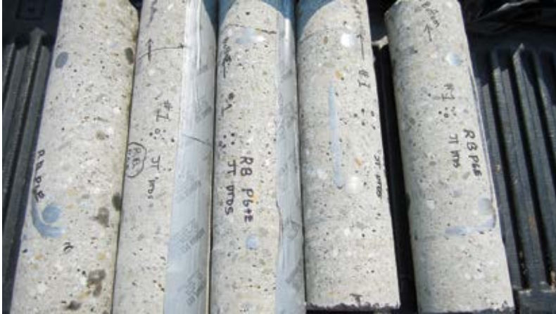
Fig. 6: Cores taken from a 24 in. (600 mm) wall that went to the testing lab for inspection
