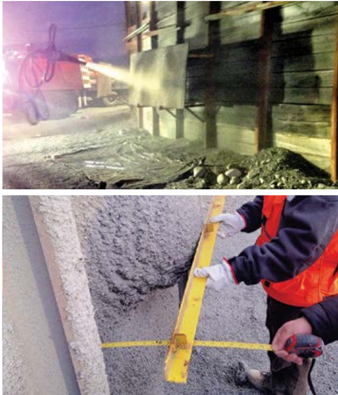
Fig. 1: The effect of pozzolanic-based rheology control agent on thickness buildup
