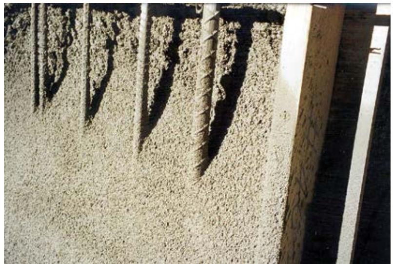
Fig. 3: Proper impact velocity and reinforcing bar encasement
