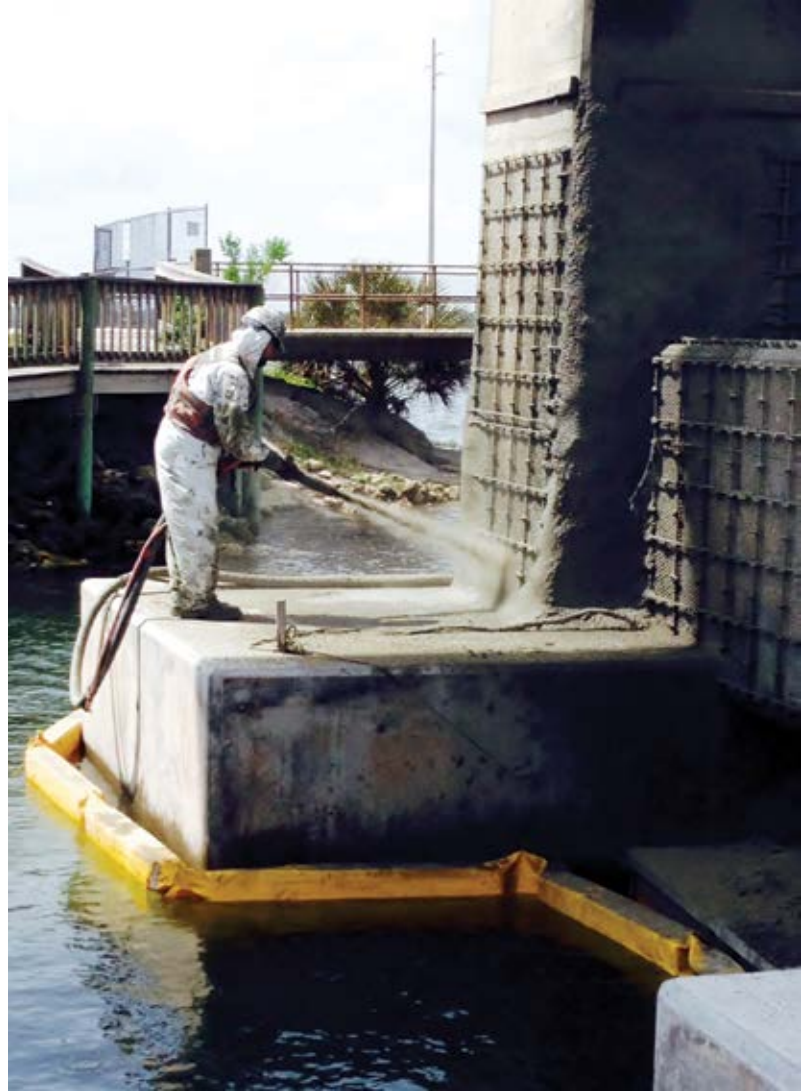
Fig. 2: Nozzleman shooting at a proper angle
