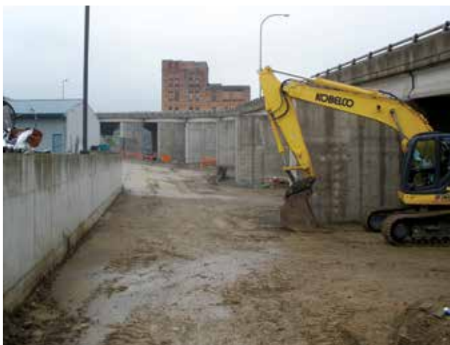
Multiple bridge piers were repaired using shotcrete with cathodic protection
